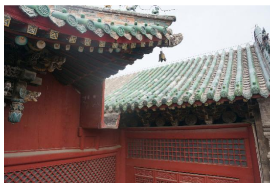
Figure 6 Joined roof with round ridge roof and gable and hip roof
