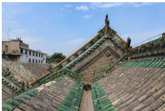
Figure 5 Joined roof with flush gable roof and round ridge roof
